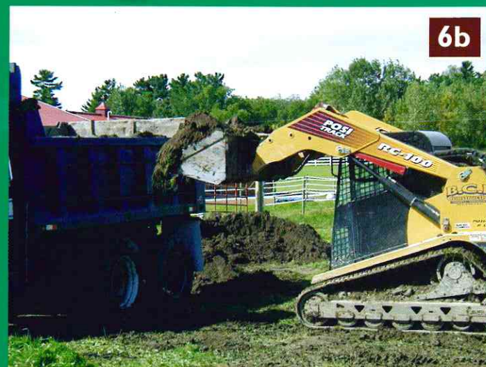
Figure 6a and b. One sunny day, Bud Carpenter (BCI Construction, Inc.) peeled away about 8 inches of compacted topsoil. The soil was stockpiled and then used elsewhere on the farm.
