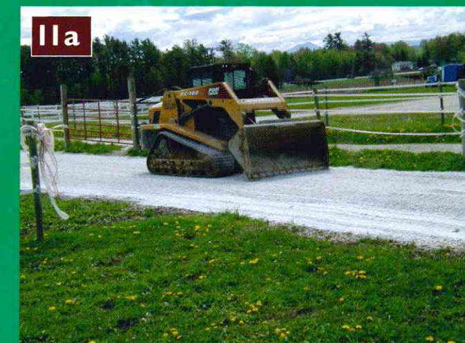
Figures 11a and b: A second layer of geotextile fabric (not shown) is rolled over the 1 1/2"-1 3/4" stone and 4" of dirty pea stone is dumped and spread on top of it. Figure 11b shows dirty pea stone (foreground) from the first paddock project that has been through a winter with horses on it. When we did the last three paddocks, we freshened up the first set of renovated paddocks. Note the weathering of a year, but still intact!
