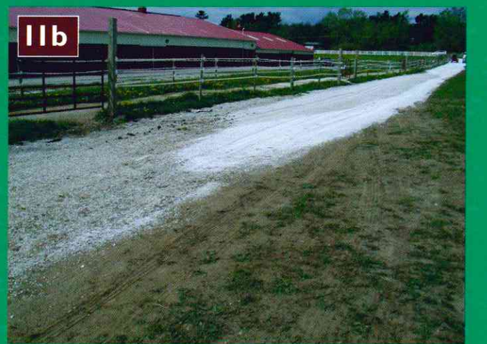
Figures 11a and b: A second layer of geotextile fabric (not shown) is rolled over the 1 1/2"-1 3/4" stone and 4" of dirty pea stone is dumped and spread on top of it. Figure 11b shows dirty pea stone (foreground) from the first paddock project that has been through a winter with horses on it. When we did the last three paddocks, we freshened up the first set of renovated paddocks. Note the weathering of a year, but still intact!
