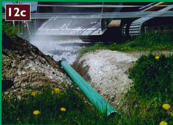
Figure 13. Water drains from the low point of the sacrifice area. Drainpipe carries water under travel lane to grassed buffer. The grass buffer filters drainage water, and some water infiltrates the soil as it passes over the grassy area. Excess water is carried away in the French drain on the far side of the buffer.
