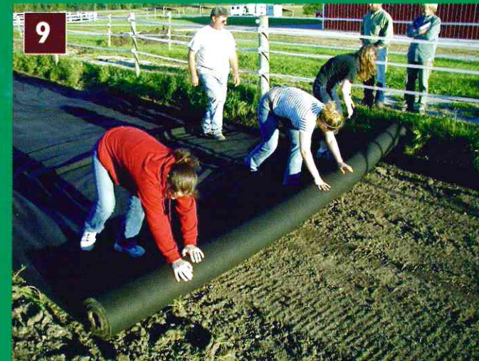
Figure 9. Horse Barn Cooperative students put some back into the work as they roll out the first layer – a sheet of geotextile.
