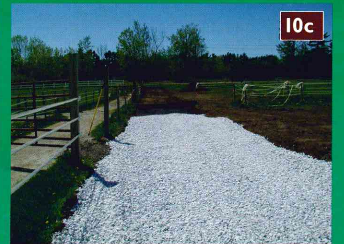
Figure 10a-c. A dump truck load of 1 1/2"-1 3/4" crushed stone is deposited and spread to a 4" thick layer.
