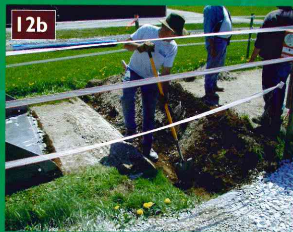
Figures 12a-d. A ditch was dug (CALL before you dig!) across the travel lane at the lowest point of each paddock, and a drainpipe was placed at a slight downward angle. The ditch was filled in with soil and topped with dirty pea stone. Crushed rock was dumped at the grass buffer end of the pipe to allow better diffusion of water as it passes through the buffer to the French drain.
