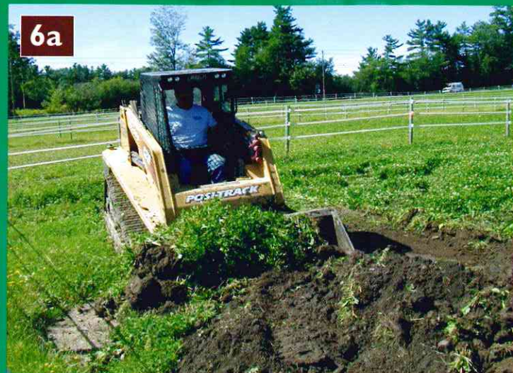
Figure 6a and b. One sunny day, Bud Carpenter (BCI Construction, Inc.) peeled away about 8 inches of compacted topsoil. The soil was stockpiled and then used elsewhere on the farm.
