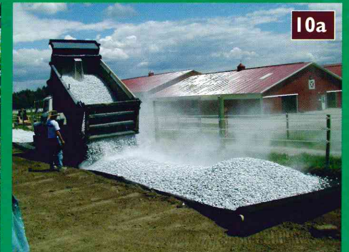
Figure 10a-c. A dump truck load of 1 1/2"-1 3/4" crushed stone is deposited and spread to a 4" thick layer.
