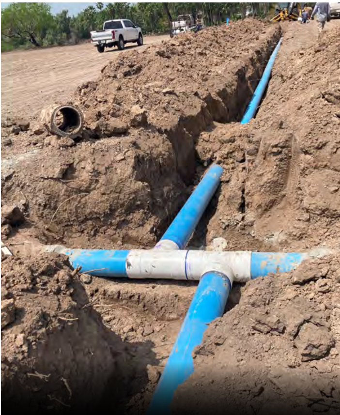
FIGURE 3.16 Irrigation Pipeline Installation in Arroyo Colorado Watershed (Source Ronnie Ramirez)
