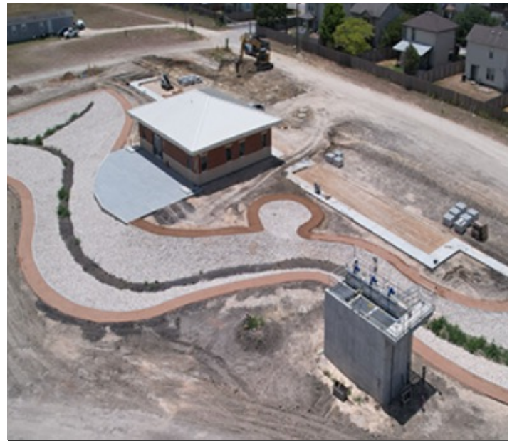
FIGURE 2.1 Vegetated Bioswale (0.36 acre) Surrounded by Crushed Granite Walkway (Source City of Kyle)
