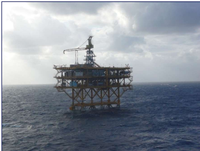
Figure 1: Walter Oil and Gas Coelacanth Fixed Platform
