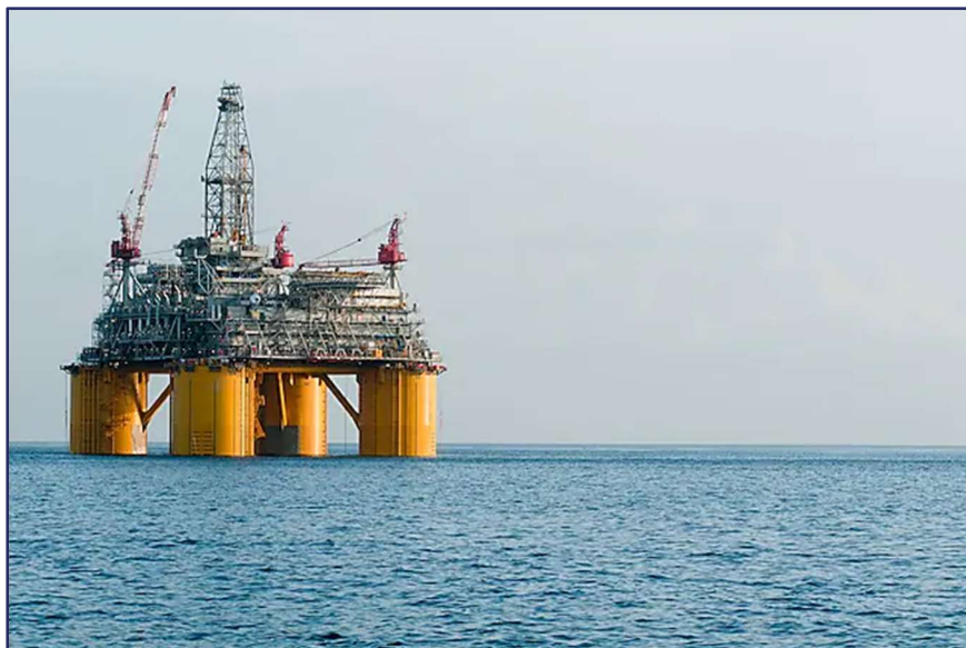
Figure 2: Shell’s Mar’s B Project / Olympus TLP Floating Production Unit
