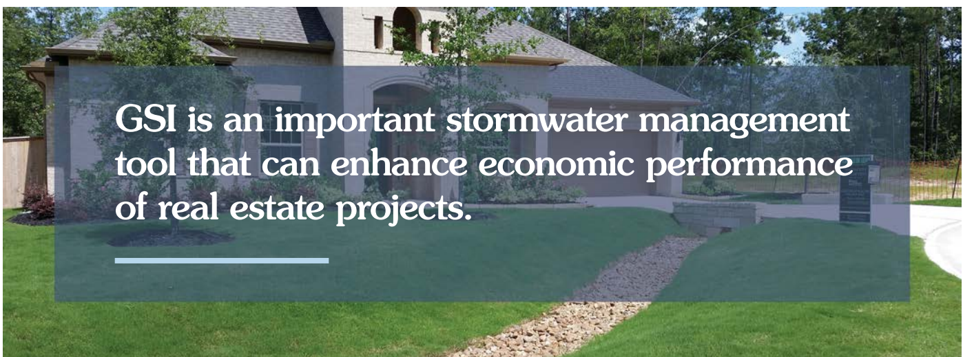
Bioswale in single-family residential development. R. G. Miller Engineers, Inc.
