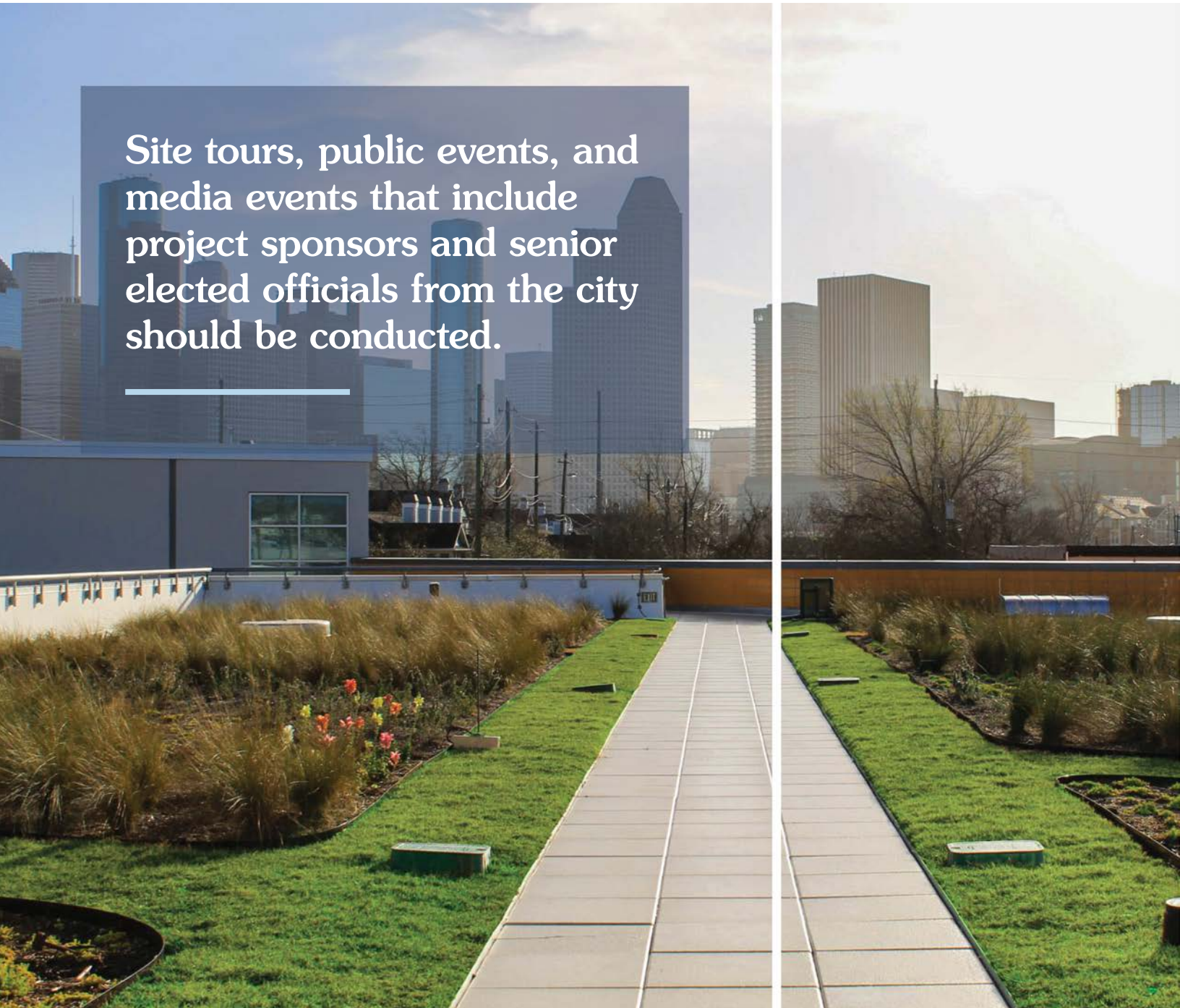
Green roof on Carnegie Vanguard High School. Asakura Robinson.
