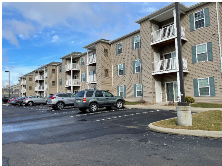
Figure A. Parking area without accessible parking or curb cuts at Parma Village Senior Apartments, Parma, Ohio.
