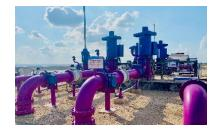
Purple pipes for reuse transmission at the Emek Hefer Water Reclamation Project facility. Photo: EPA.
