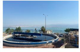
View of the clarifier at the Ein Bokek treatment and reuse facilities. *Photo: EPA.*
