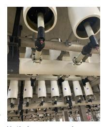
Vertical reverse osmosis technology is a space-efficient treatment option in use at the Sorek Desalination Plant. *Photo: EPA.*
