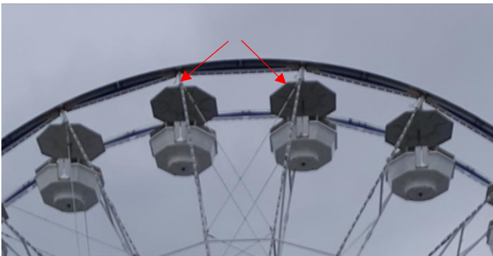
Fig. 3 and Fig. 4 – Tie rod connection points not easily accessible by patrons.
