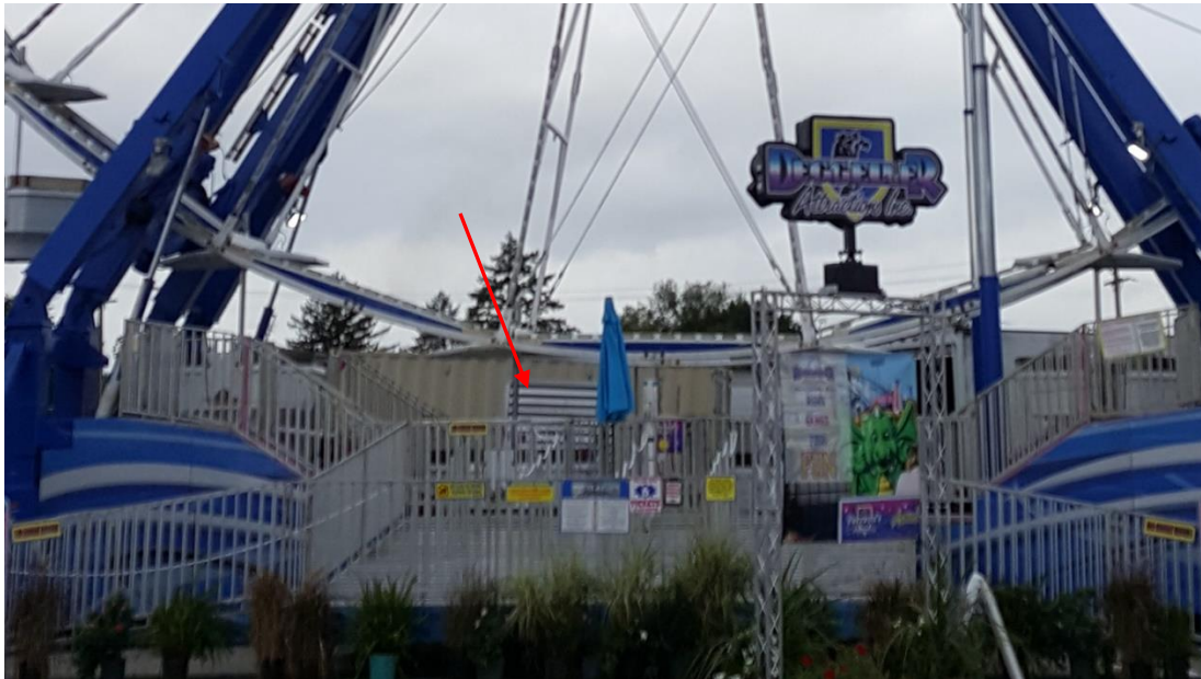
Fig. 9 – Notes the location and proximity of the power plant to the Wheel. The slats shown are to let air into the power plant but also do little to muffle the noise of the power plant
