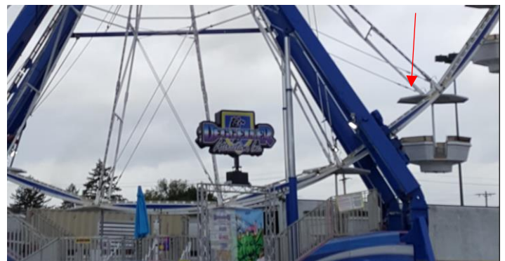
Fig. 3 and Fig. 4 – Tie rod connection points not easily accessible by patrons.
