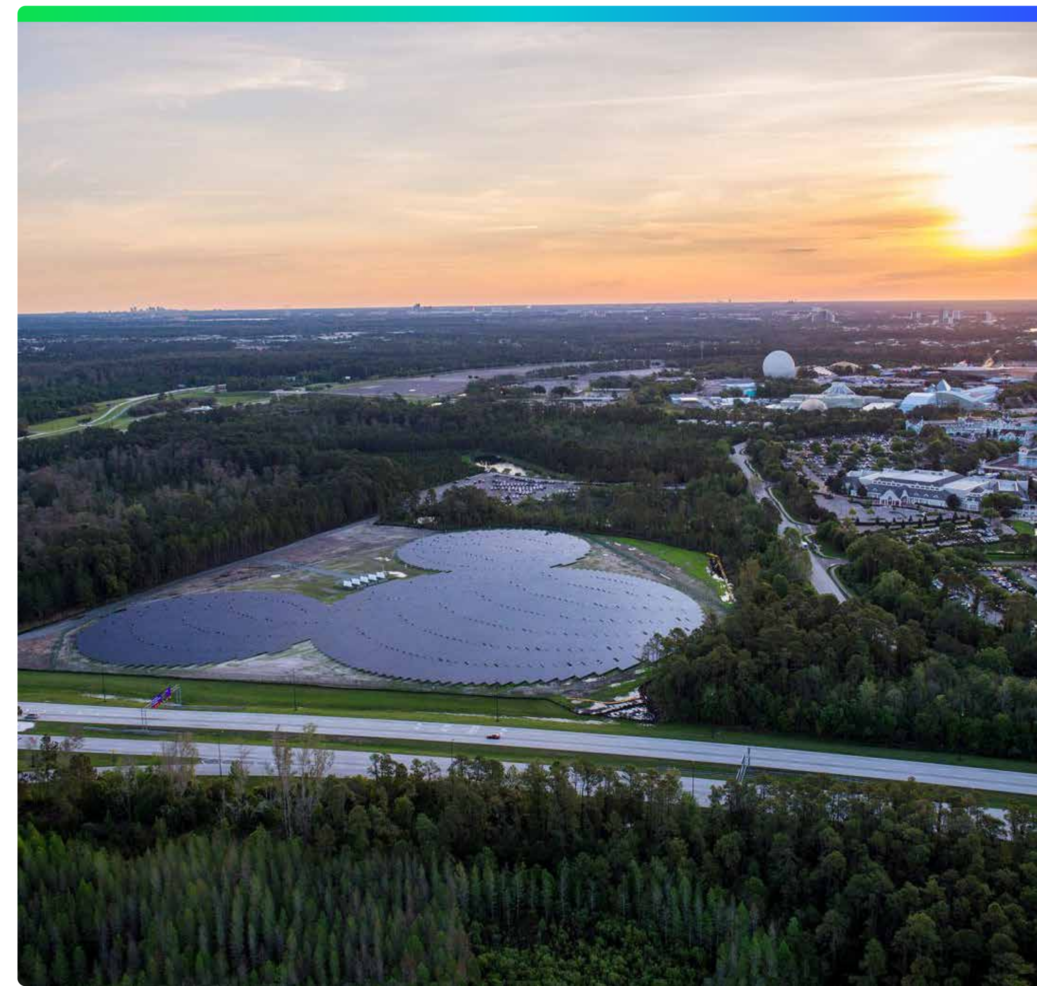
Mickey-shaped solar facility (located near EPCOT), which provides power to Walt Disney World, was built in partnership with Reedy Creek Improvement District and Duke Energy.
