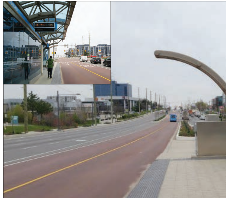
Figure 2-39. Examples of a Viva far side median stop, located immediately after an intersection to accommodate left-turn lanes for motorists
