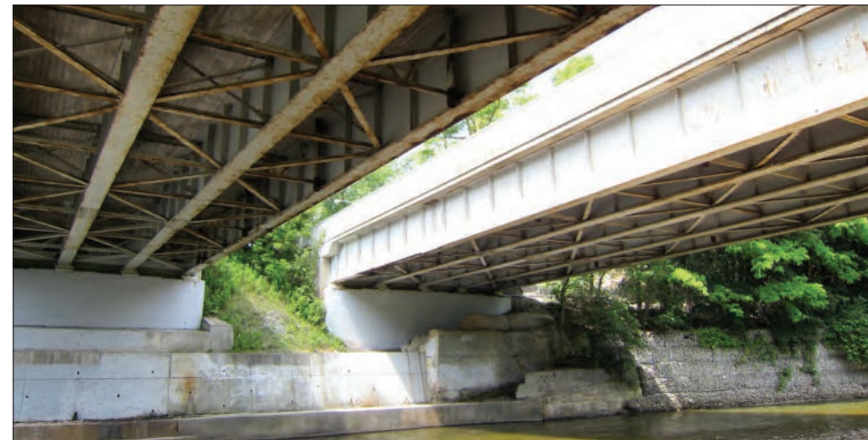
Figure 2-25. Credit River Bridges
