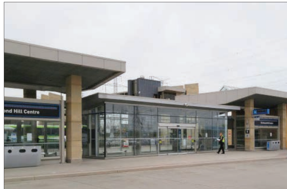
Figure 2-36. Transit terminal (Richmond Hill Centre Terminal) served by York Region Transit, Viva, and GO Transit buses and connected to Langstaff GO Station (commuter rail)
