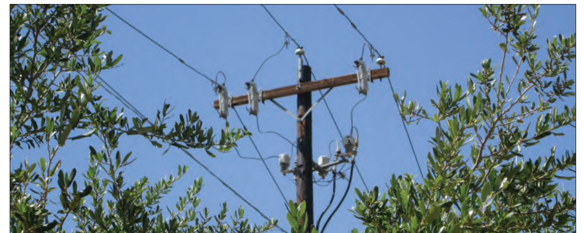
Figure 5-77. Trees and hydro wires
