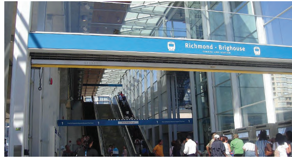
Figure 2-42. Richmond-Brighthouse Station, the southern terminus of the Canada Line in Richmond BC
