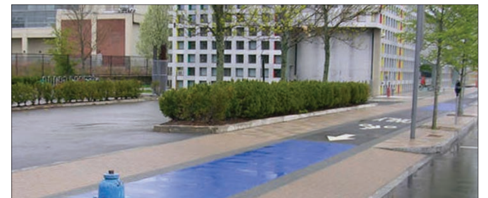
Figure 5-54. Raised cycle track
