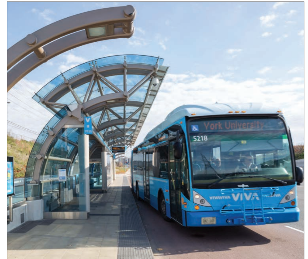
Figure 2-40. Example of a Viva nearside median stop, located immediately before an intersection
