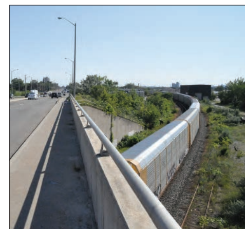
Figure 2-26. Dundas Street over the CP Rail and GO Milton Line corridor
