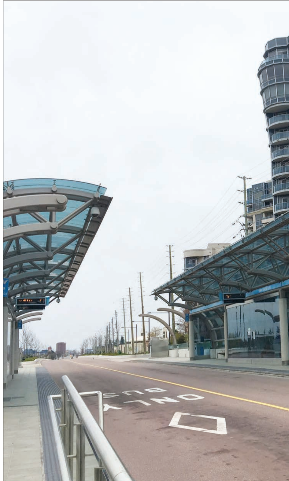
Figure 2-38. Viva's median-running, dedicated transitways
