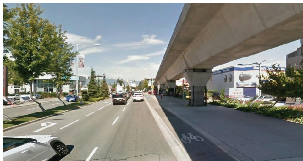
Figure 2-41. No. 3 Road with street oriented retail, median landscaping, cycling lanes and the elevated guideway
