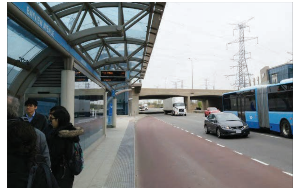
Figure 2-37. Bayview BRT Station at Highway 7 and Bayview Avenue
