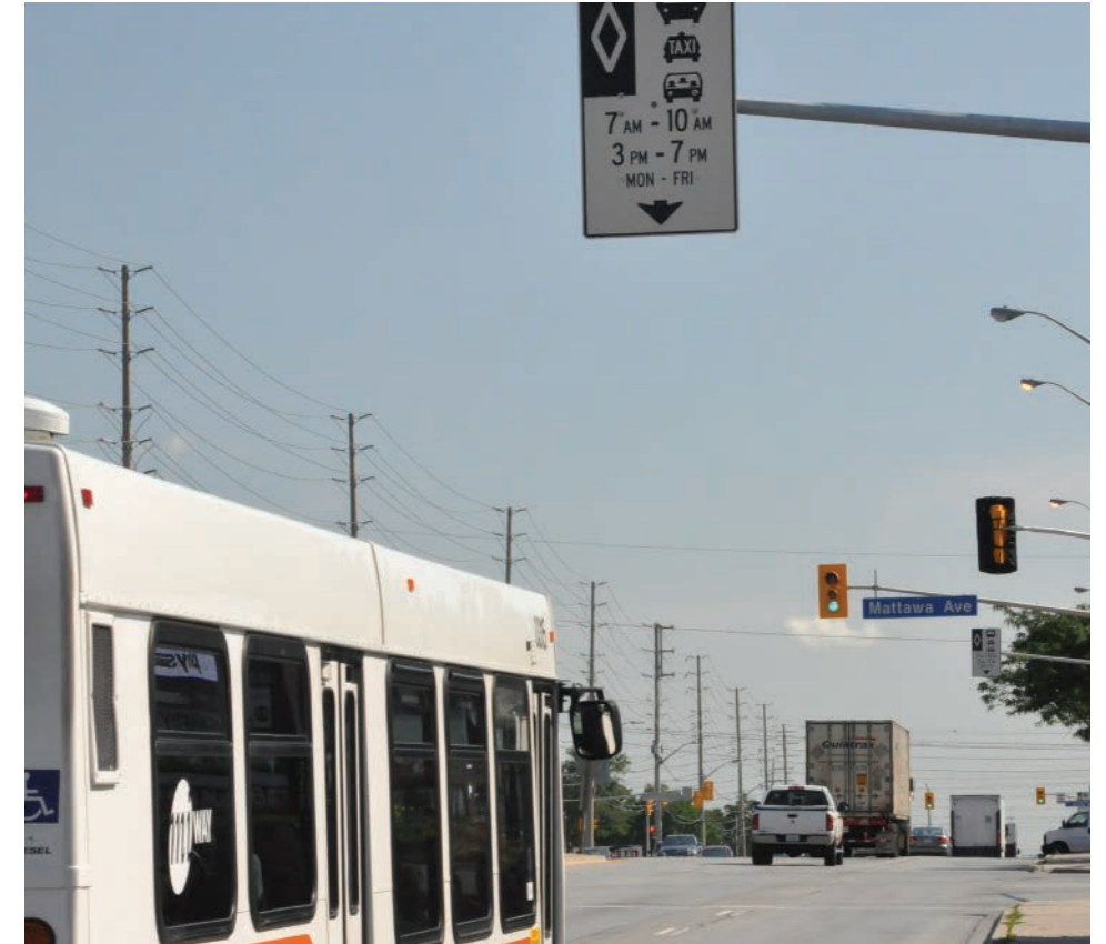
Figure 2-16. Dundas Street HOV Lane at Mattawa Avenue
