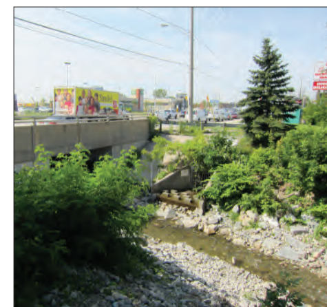
Figure 2-27. Dundas Street over Little Etobicoke Creek
