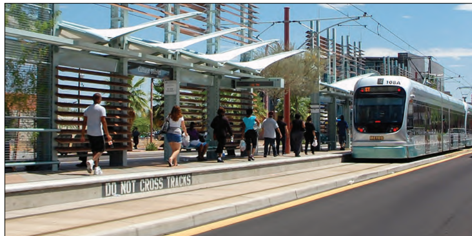
Figure 4-6. Valley Metro Light Rail, Phoenix, Arizona
