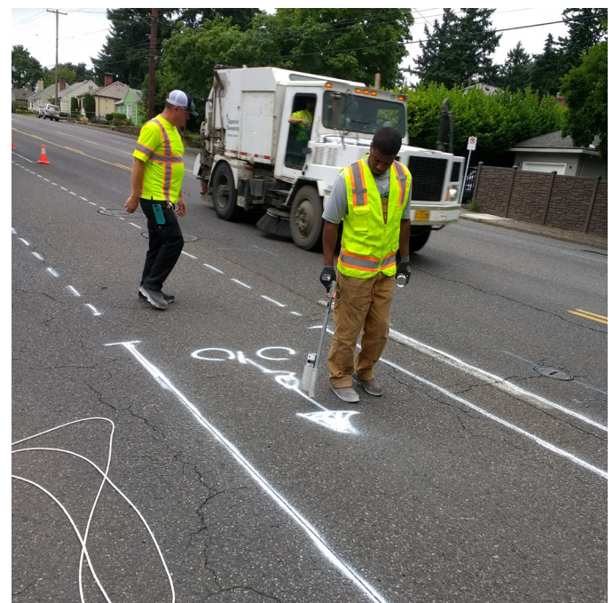
PBOT crews painting layout lines on NE 102nd Ave.
