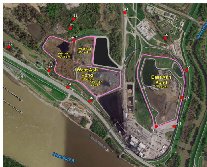
WOOD RIVER COAL ASH PONDS
