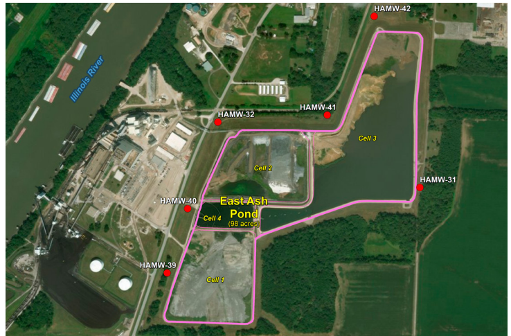
HAVANA COAL ASH POND
