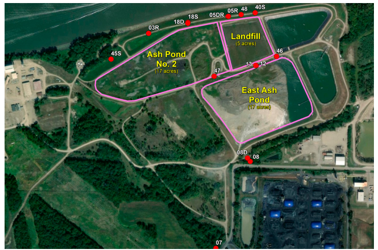
HENNEPIN EAST COAL ASH PONDS
