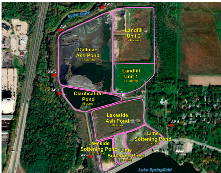
DALLMAN COAL ASH PONDS AND LANDFILL
