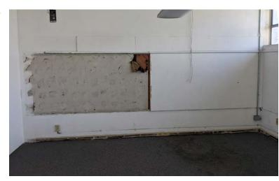
Interior walls are gypsum board/plaster. Walls have signifacant damage and uneven texture. Existing conduit and recptacles are surface mounted.
