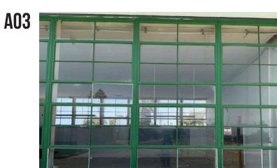
Windows are steel frame with a single pane glass throughout the facility. The steel frame is galvanized and seems to be in good condition, but some opening devices are not functioning. Paint on window frames is lead based.
