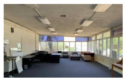
Ceilings are tiles adhered to joists in classrooms, plaster ceiling in enclosed NE office space and other office areas. The ceiling tiles are in poor condition with stains of water intrusion from the roof. The plaster ceiling was intended as an exterior covered walkway and is not appropriate for interior space.
