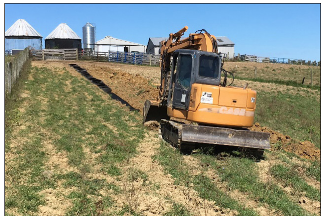
Figure 3. A backhoe creates a trench for the all-weather path.
