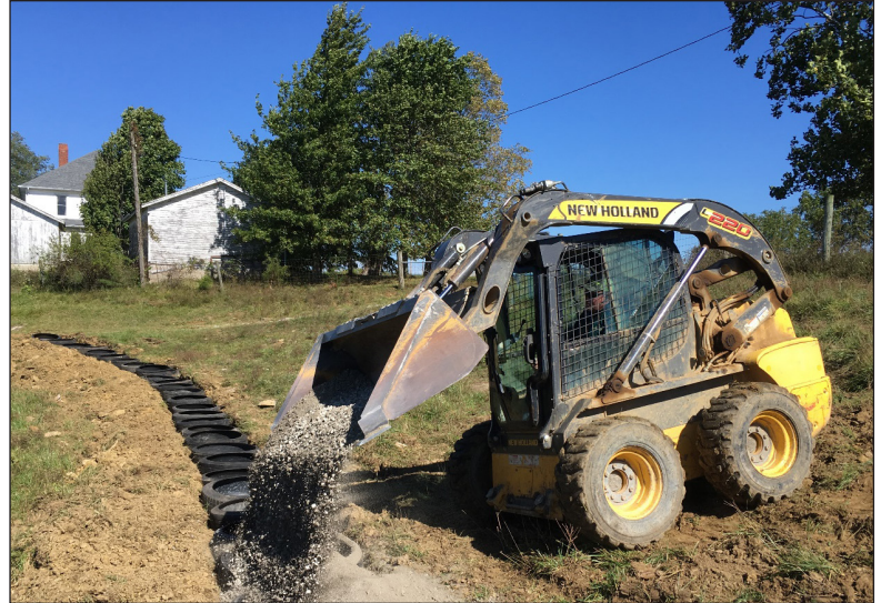
Figure 5. The tread cylinders are filled with rock.
