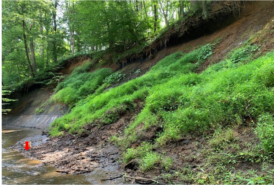
Figure 5. POI-2: Exposure just east of Boundary Road at Big Brook, Colts Neck, NJ. The red arrow points to a bucket that indicates the approximate location of this cliff in the 1970’s as remembered by J. Brown. It gives an idea of the degree of erosion and why study of Coastal Plain exposures are so challenging. The area above the arrow is highlighted in Figure 6. Photo facing southeast; by Justin Andell, RVCC.
